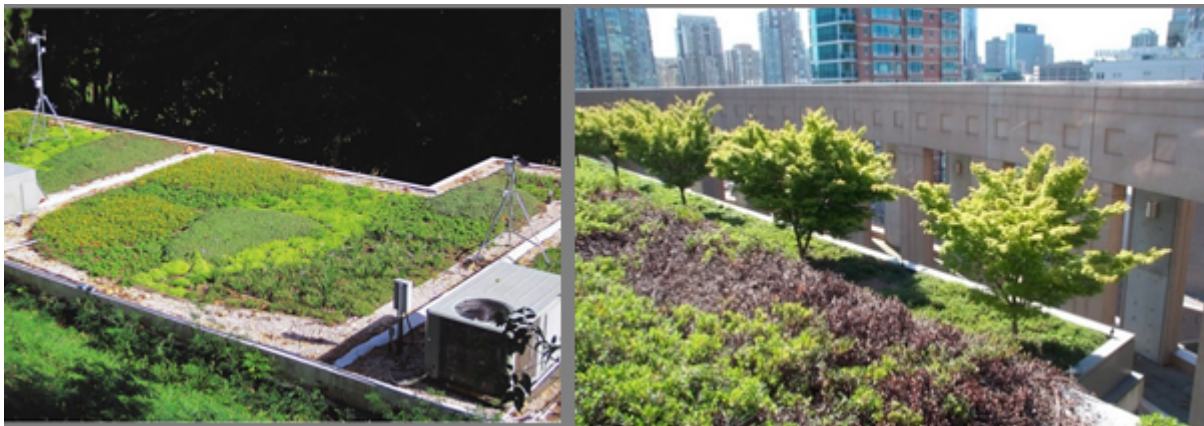
Figure 2. Extensive green roof at International Institute of Tropical Forestry in San Juan, Puerto Rico (left); Intensive green roof at the Vancouver Public Library (right).
