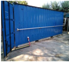
Figure 82: External air duct for outdoor testing
