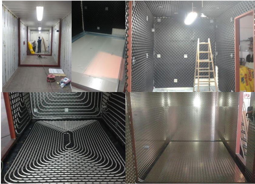
Figure 43: Assembly process of the test rooms
