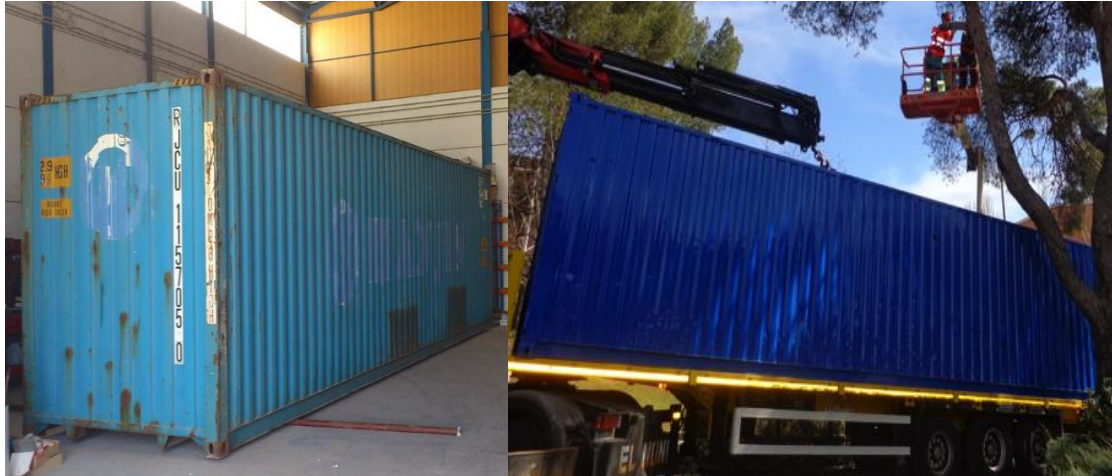
Figure 38: Container before and after exterior paint application
