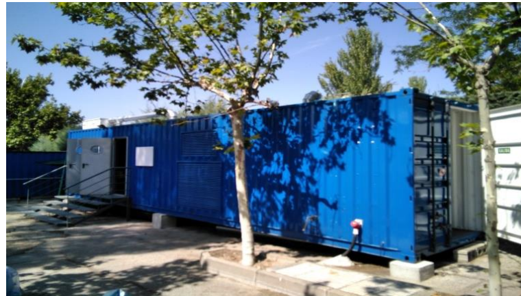
Figure 54: Entrance door to the Control Room on the right side of the Test and Control Container
