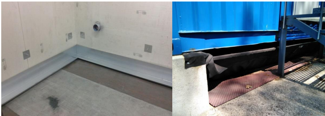
Figure 44: Pool for the collection of waste or liquid released during the performance of tests
