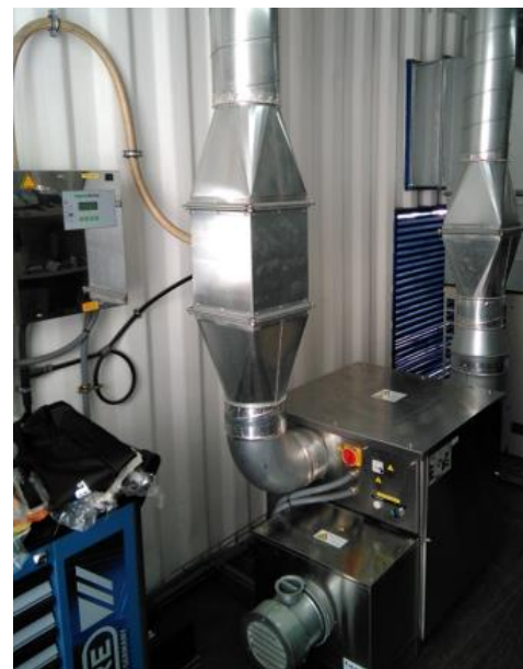
Figure 59: Humidifier/dehumidifier
