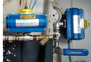
Figure 79: Filling and venting water valves
