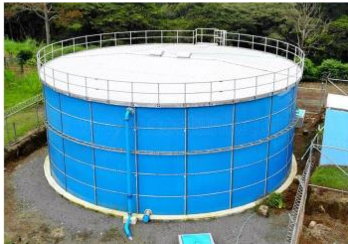
Fig.3 Reactor de digestión anaerobio UASB (Upflow Anaerobic Sludge Blanket)
