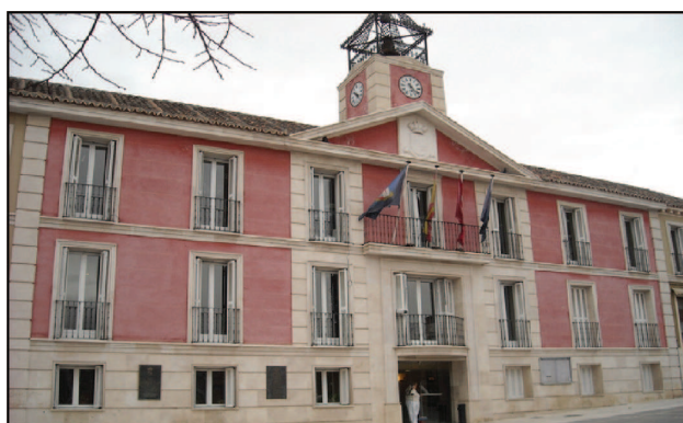
Figure 6. Real heritage (down) through AR in Aranjuez.
