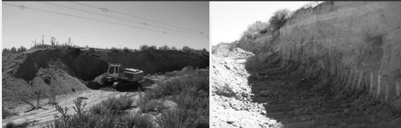
Figure 5 Left: Backhoe preparing a vertical face for sand martins at an inactive extraction face. Right: Final result. Source: Zoë Rohrer (LafargeHolcim).
