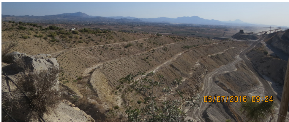
Figure 6.3 Example of a restoration that involved decreasing slopes by refilling with material.
