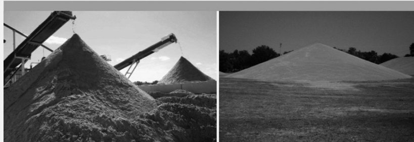
Figure 3 Active stocks without vertical faces. Both stockpiles dissuade sand martins from making burrows in them. Source: FlickrCommons.
