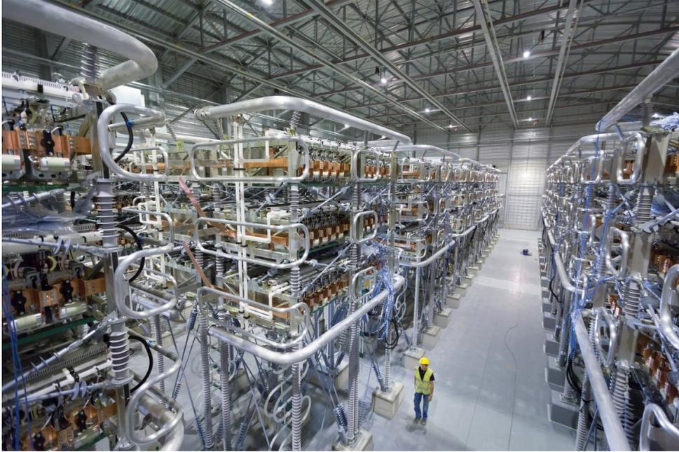
Figure 2.1: Converter hall of a 1000 MW HVDC transmission link between France and Spain. [5]
