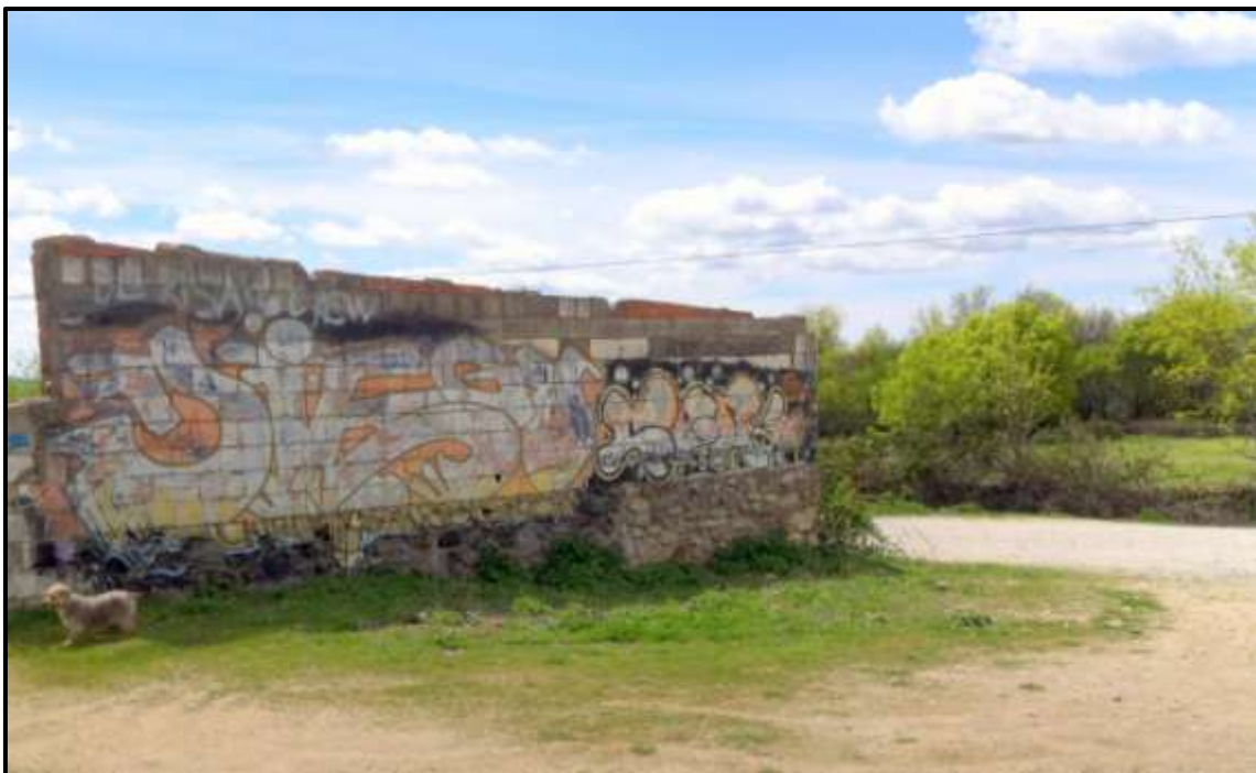
Fig. 47 . Photograph of a wall of an abandoned building in the country side used as a canvas for graffiti. Graffiti and skate parks are a continual source of conflict with the young. The first is seen as an act of vandalism and the second as one of noise. (Photograph by author)
