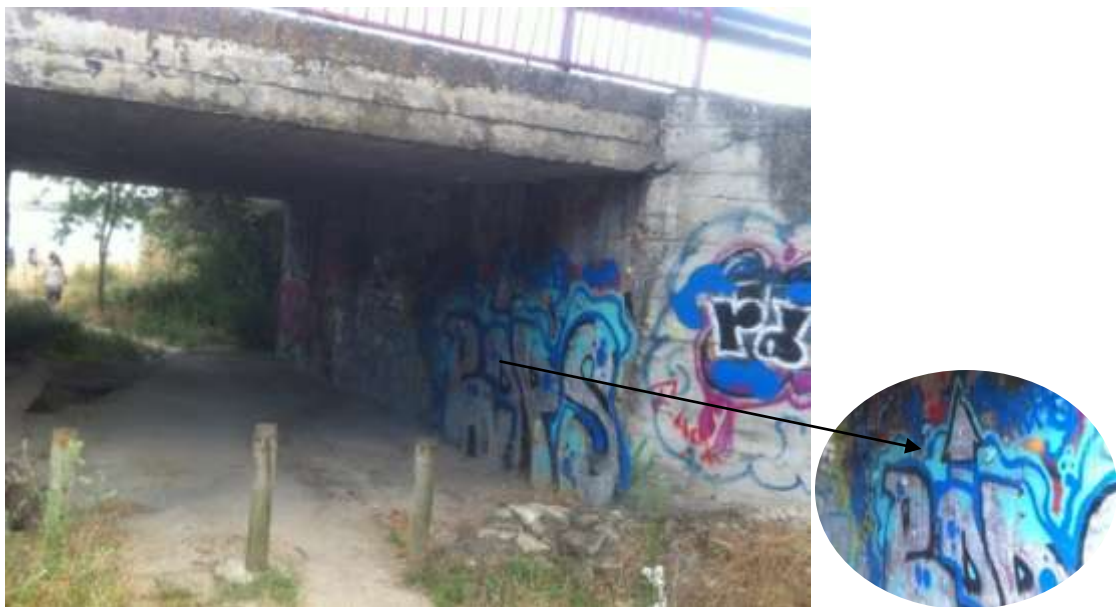
Fig.185. Photograph of a secret meeting place under a bridge; a space which teenagers have carved out for themselves to shelter from the cold and sun and meet up. The wall has climbing points which the kids who use this hide out here have they themselves attached to it. (Photograph by M. Ramon)
