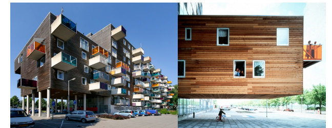
Figura 17. WoZoCo Apartament Building, MVRDV
