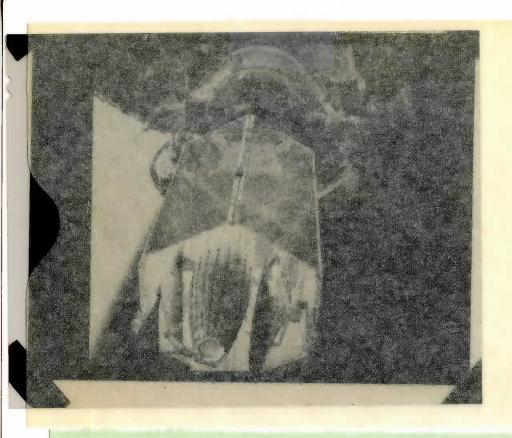
SATELLITE DEPLOYMENT -- The 18.5-ton Tracking and Data Relay Satellite (TDRS) is elevated upward in preparation for deployment from the cargo bay of Discovery. The new TDRS and a similar satellite launched in 1983 expand U.S. space-based signal relay coverage to 85 per cent of the globe for equatorial orbits.
