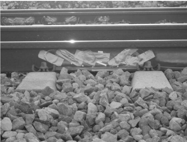
Fig. 2. A section between sleepers covered and protected.
