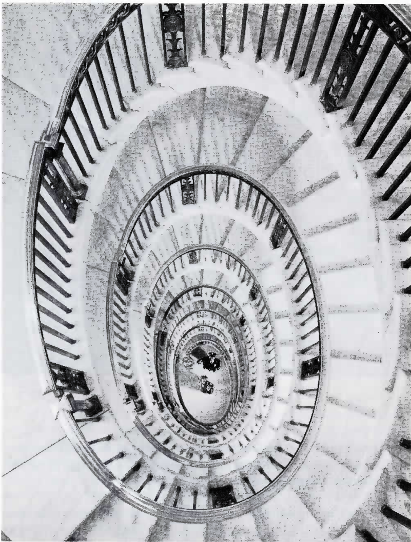
Two self-supporting elliptical spiral staircases constructed of marble and bronze connect five stories. Few others exist in the world. The Paris Opera, the Vatican and the Minnesota State Capitol are among those with similar structures.
