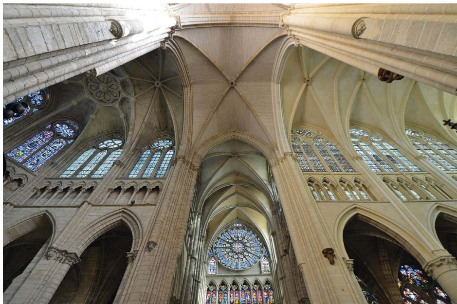
Fig. 5. Châlons-en-Champagne cathedral, crossing, looking south, c. 1240s-1260s (Photo: Tom Nickson).
