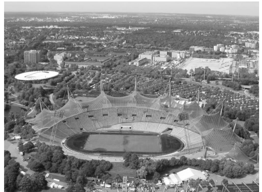
Imagen 72. Mark, Laura. "Six projects by Pritzker winner Frei Otto." The Architects Journal , 11 Mar. 2015
