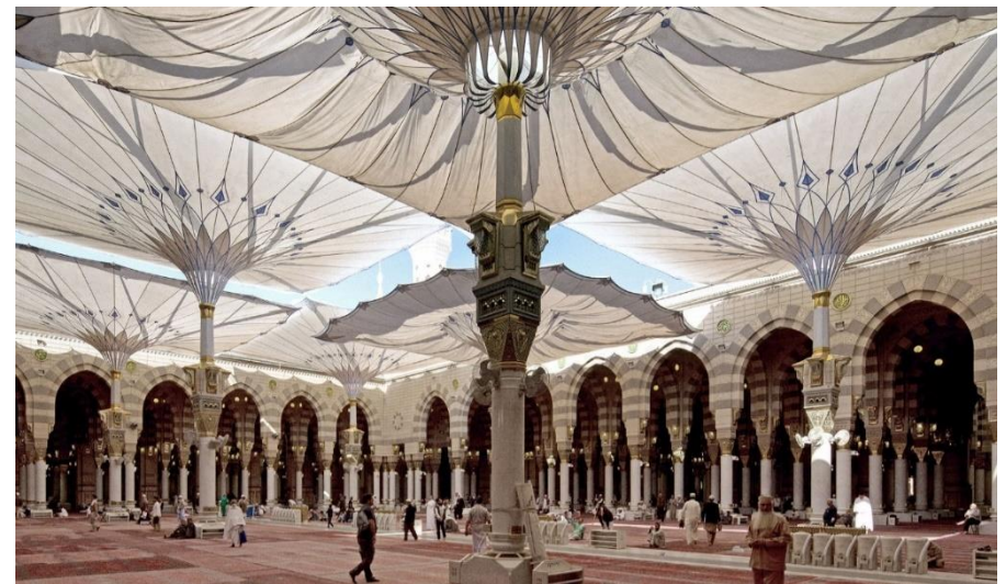
Imagen 17. Convertible shading roof for the Prophet's Mosque in Medina, Saudi Arabia, SL Rasch. ( https://www.sl-rasch.com/en/projects/courtyard/ )
