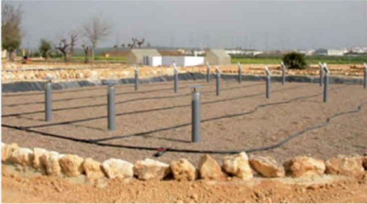
Figure 1-4: Water distribution in a vertical flow constructed wetland at the research centre CENTA, Carrión de los Céspedes, Sevilla, Spain. From: (Ortega et al., 2010).
