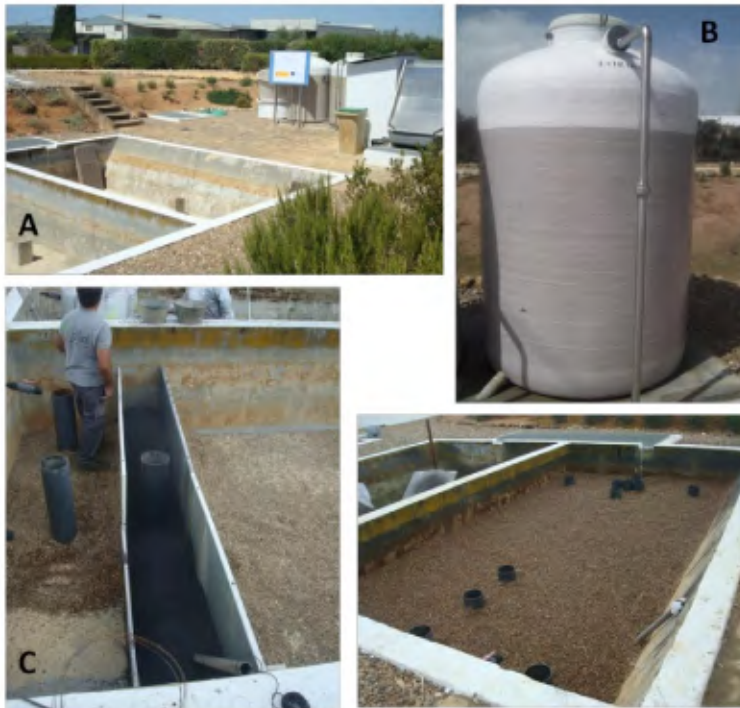
Picture S 4-1: Photographs of the construction of the METland in CENTA, Carrión de los Céspedes, Sevilla. A) A peat filter pool in misuse was emptied and reused to install the METland; B) Imhoff tank; C) Construction of the conductive bed; D) General view of the METland just completed.
