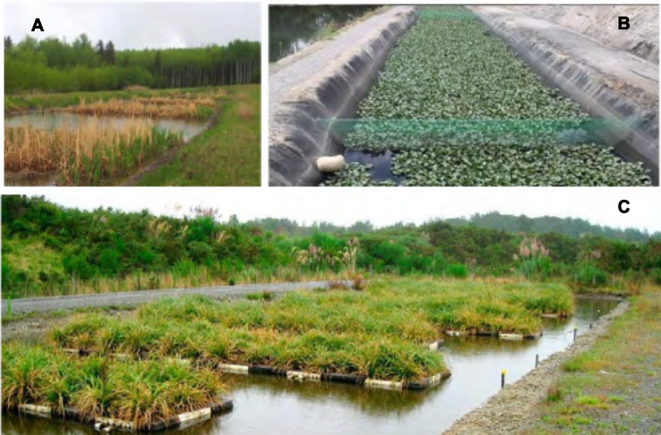
Figure 1-2: Pictures of different surface flow constructed wetlands. A: Free Water Surface (FWS) at Knockholt Landfill, Region of Bulckley/Nechako, Houston, BC; B: Free Floating Macrophyte (FFM) C: Floating Emergent Macrophyte (FEM).
