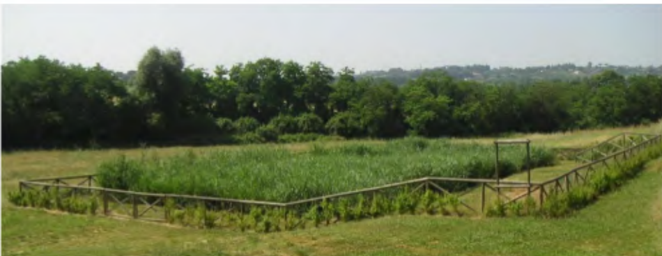
Figure 1-3: An example of a subsurface flow constructed wetland to treat urban wastewater for 362 p.e. in Ondrejov, Czech Republic.
