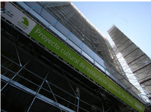
Fig. 12. The lift platform for the public that permitted to visit the restoration works on the façade
