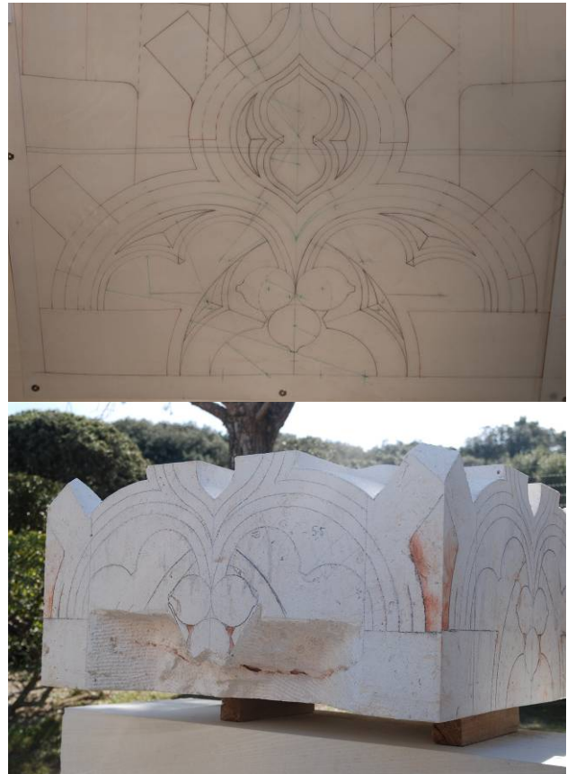
Fig. 10. Pinnacle detail hand drawing in 2D and the same drawing on the stone to be sculpted
