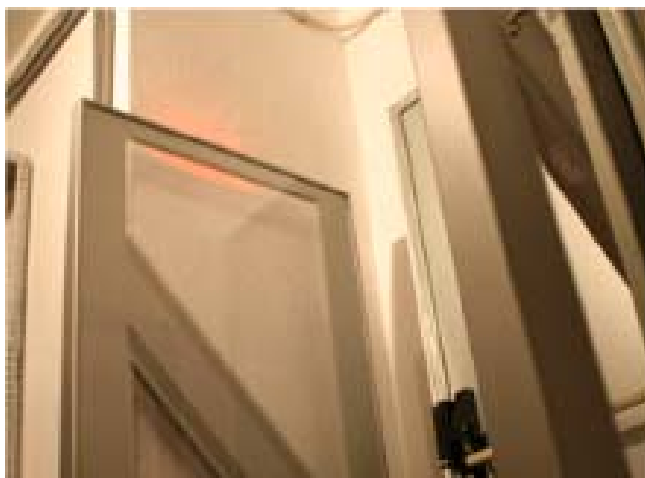
Figure 4. Gate Subsystem deployed in a vault.
